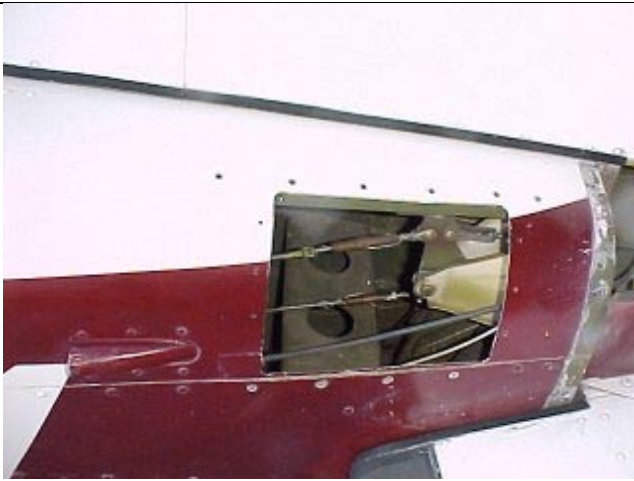
Completed access hole on left (port) side
